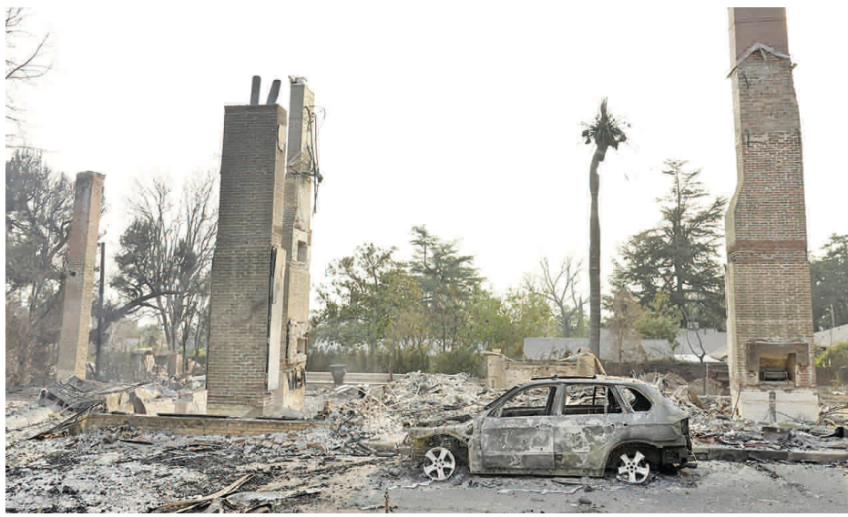
The Andrew McNally House, built in 1887 by the co-founder of the Rand McNally publishing company, is pictured after it was destroyed by the Eaton Fire, Thursday, Jan. 9, 2025, in Altadena, Calif. (AP PHOTO/CHRIS PIZZELLO)
