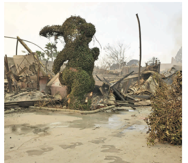
A welcome path leads to the charred remains of the Bunny Museum, Thursday, Jan. 9, 2025, in Altadena, Calif. (AP PHOTO/CHRIS PIZZELLO)
