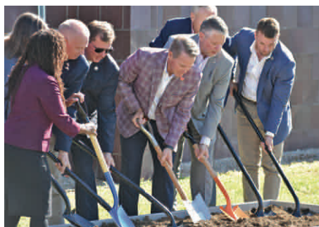
Participating in a groundbreaking ceremony Thursday, Oct. 3, for the Transportation Research Center’s new Impact Laboratory were, from left, TRC Board Chair and OSU Engineering Dean Ayanna Howard, Rep. Tracy Richardson, Rep. Tim Barhorst, House Speaker Jason Stephens, Ohio Lt. Governor Jon Husted, TRC President Brett Roubinek, Senator Bill Reineke and Rep. Jay Edwards, who serves as the Ohio House finance committee chairperson. (TRC PHOTO)
