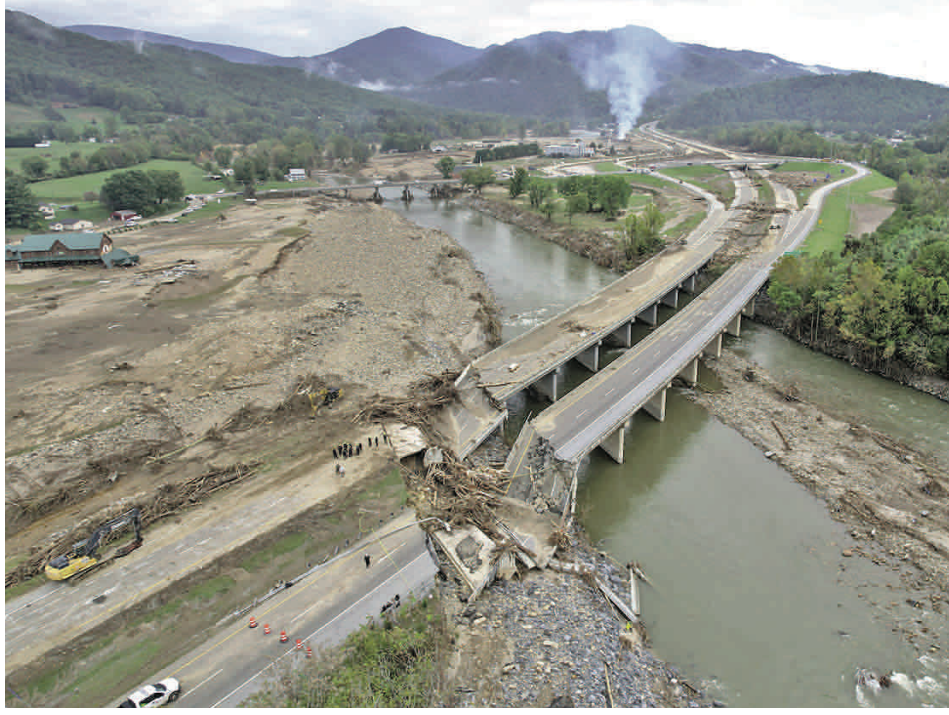
A bridge along Interstate 26 is destroyed in the aftermath of Hurricane Helene Friday, Oct. 4, 2024, in Erwin, Tenn. (AP PHOTO/JEFF ROBERSON)
